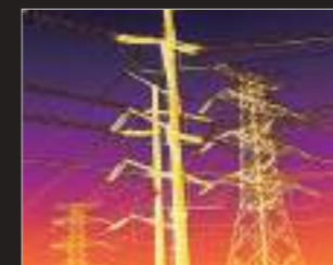
Electric Routine Inspection
